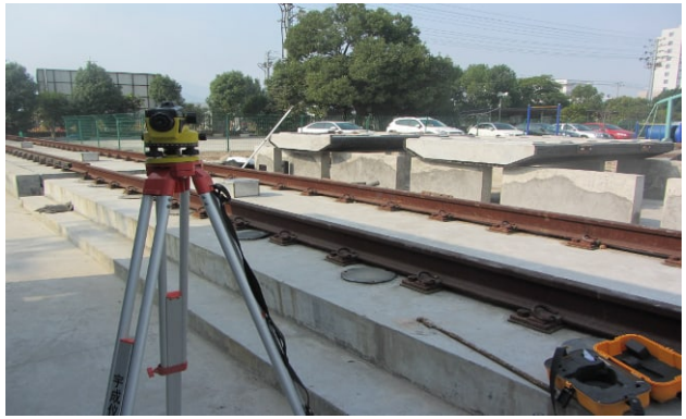
Tiantie on-site testing
