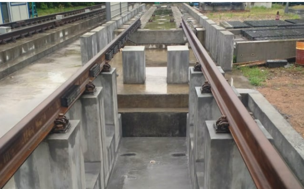
Tiantie on-site testing
