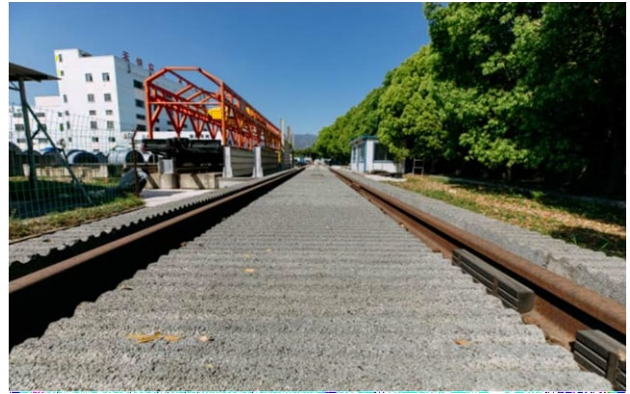
Tiantie on-site testing
