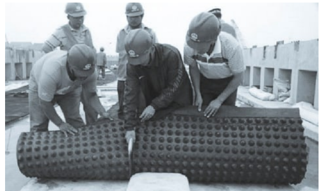
Installation of Track Mats
