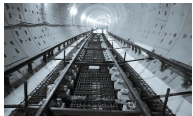
FST on Helical Steel Springs: Kunming Metro
