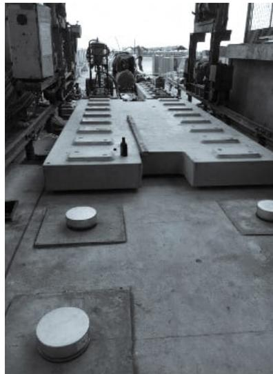
FST on Rubber Bearings: Ningbo Fenghua Line
