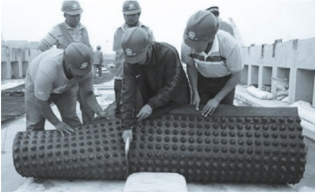
Installation of Track Mats
