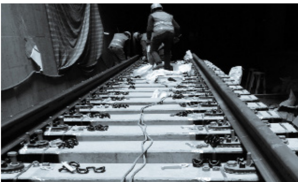
Installation of Sleeper Boots
