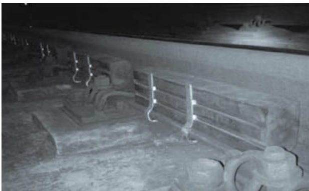
Installed Rail Dampers
