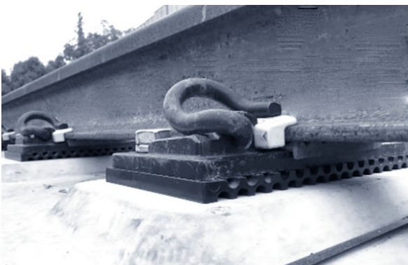
Installed Rail Pads
