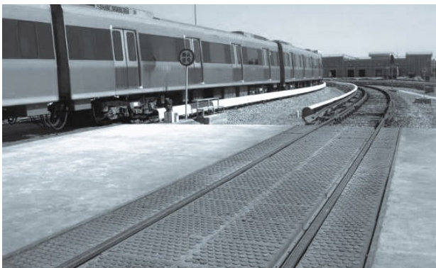
Tiantie Level Crossing System: Beijing Olympic Park
